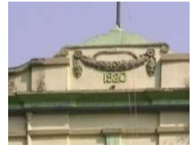
Stucco script on building
