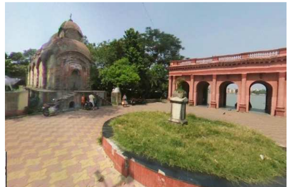
Showing Signs of Deterioration
