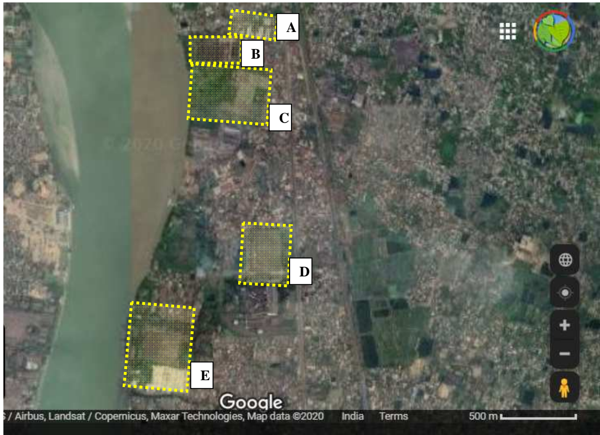
[A] Empire Jute mill; [B] Kelvin Jute mill; [C] Kinnison Jute mill; [D] Titagarh jute mill no.2; [E] Titagarh jute mill / National Jute Manufactures Corporation Ltd. (NJMC)
