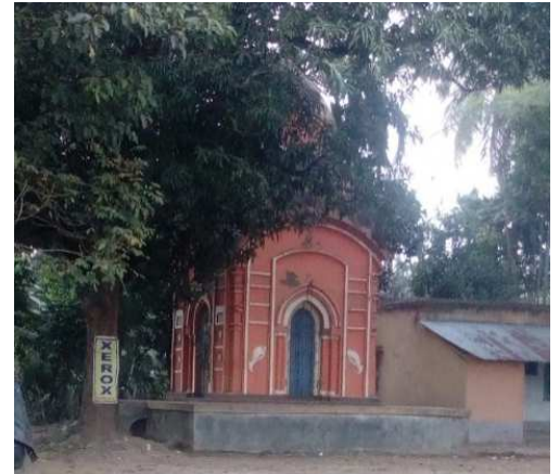
View from S-E corner
